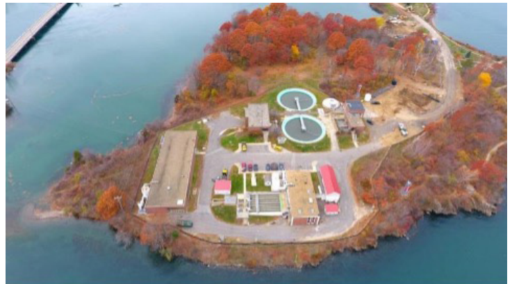
Aerial view of the WWTF shortly after construction began
