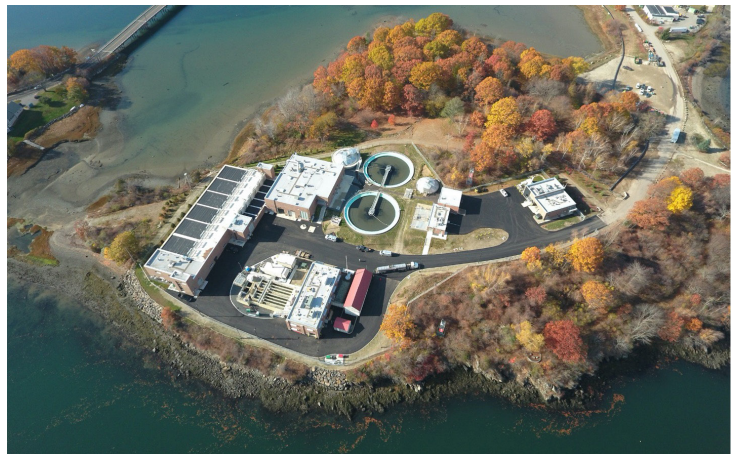
Aerial view of the WWTF after construction
